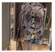
Poor installation becomes worse over time and faults accumulate. A typical installation is shown here. The low IP rating of the components also contributes to this high fault rate. Hardened connectors would avoid this problem.
